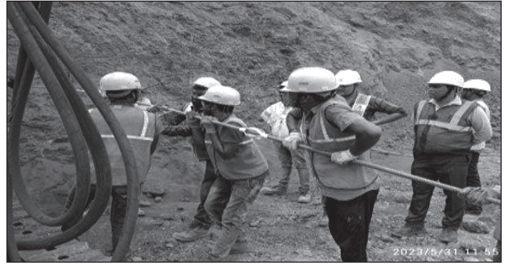
(Figure-02 : Nail installation)
